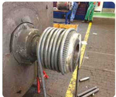
Heating a coupling for dismounting
